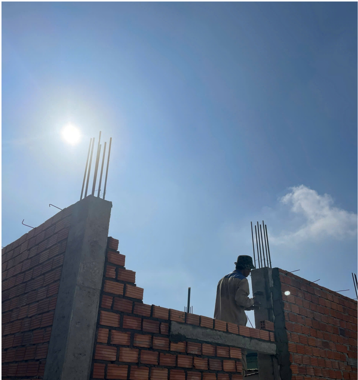
An outdoor worker labouring in extreme heat at a construction site in Binh Tan District, May 2024. © SocialLife Research Institute, 2024
